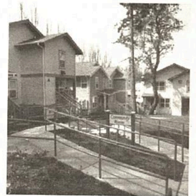
The Aki Kurose Apartments, for low-income families, built by the Low Income Housing Institute.
