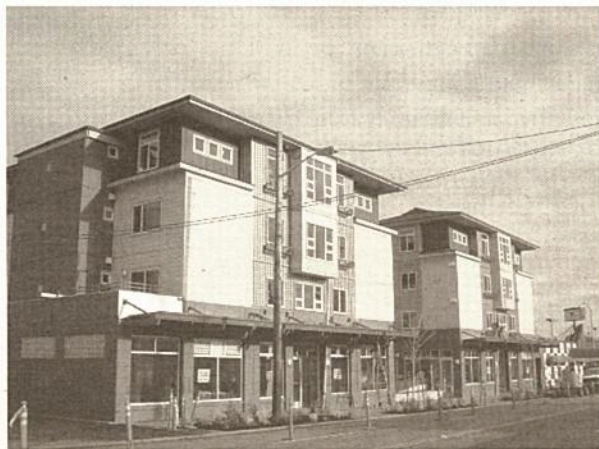
THE GREENWOOD NEIGHBORHOOD'S NEW CATE APARTMENTS. PHOTO COURTESY LIHI.
